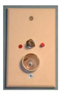
Warning: Do not connect high current devices to 12 Volt receptacle. Maximum current rating of this receptacle is: 7.5 Amps at 12 Volt DC. power supply; the other end of the coax to the connector in the rear of the cable plate.
